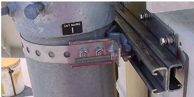
Figure C-16. Pipe Blocks
