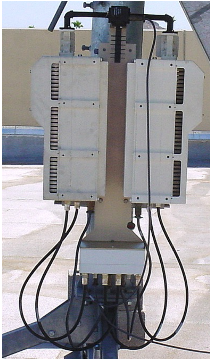
Figure B-14. Redundant Configuration
