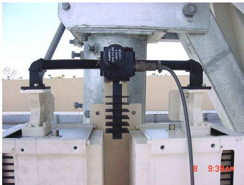
Figure B-20. Installation of the Waveguide Switch.
