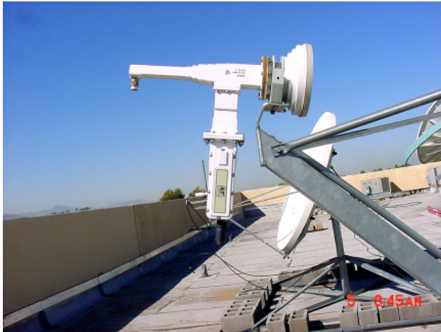
Figure 8-5. Installation of Single-Thread LNA
