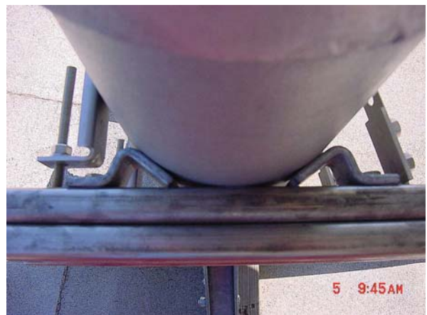
Figure C-17. Looking down at Pipe Blocks
