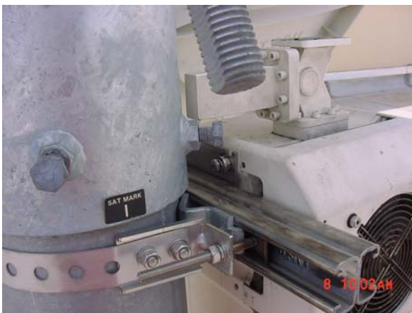
Figure B-4. Installing the Pole Bracket
