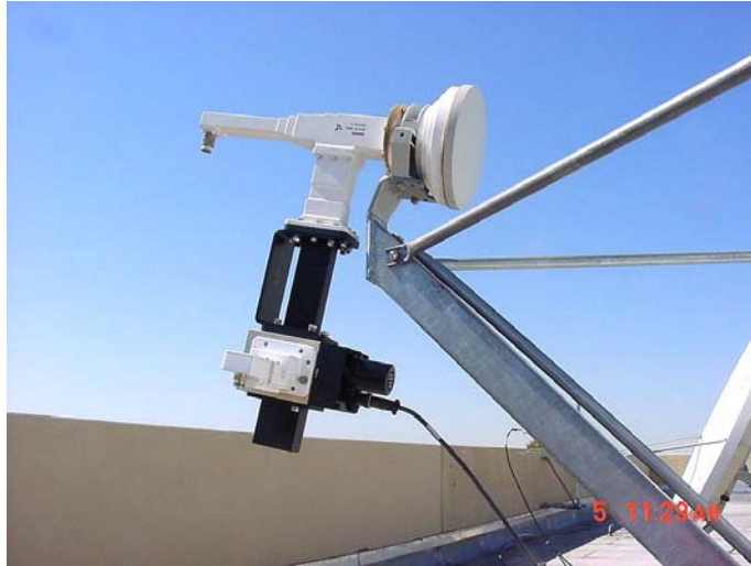
Figure 8-6. Installation of the Redundant LNA Assembly.
