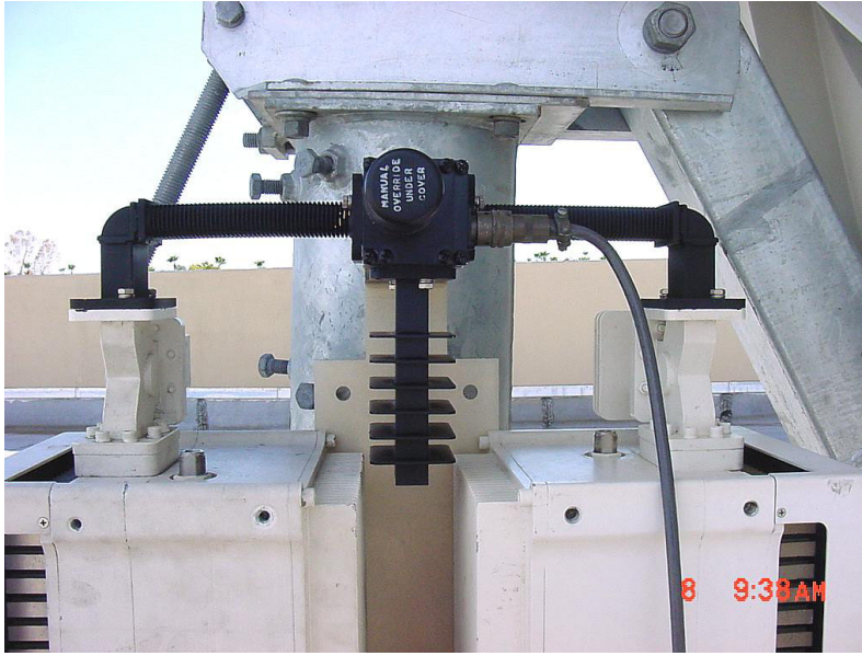
Figure 2-25. Installation of the Waveguide Switch.
