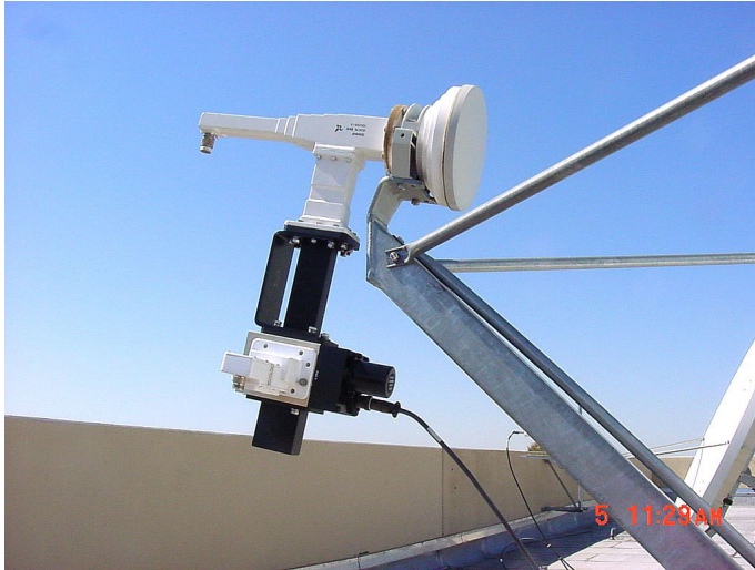
Figure 2-26. Installation of the Redundant LNA Assembly.
