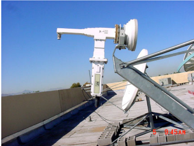
Figure 2-8. Installation of LNA
