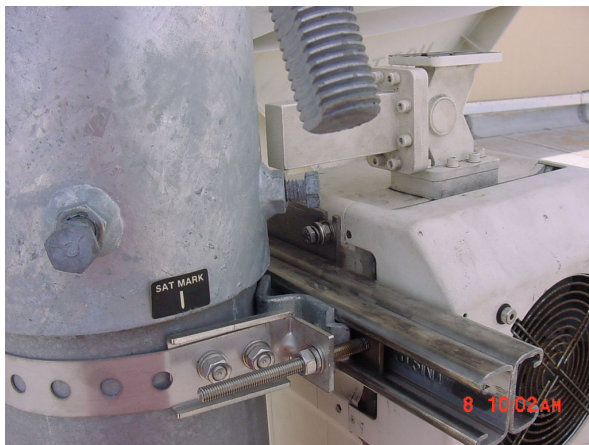
Figure 2-5a. Installing the Pole Bracket
