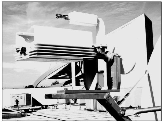
Figure 6-6. Installing the SSPA
