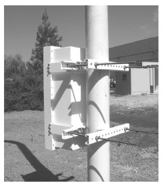
Figure 6-4. Rear View of Converter Installed on Round Pole
