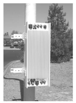
Figure 6-5. Front View of Converter Installed on Round Pole
