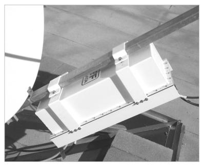
Figure 6-2. Typical Converter Unit Installation on Spar
