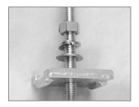
e. One threaded rod at a time, hold the washers and plate in place on the rod, and screw the rod into a spring nut, as illustrated.
