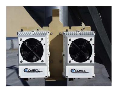
Figure A-19. Installation of XSAT Transceivers
