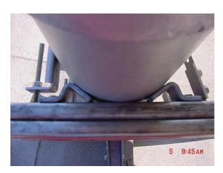
Figure B-21. Looking down at Pipe Blocks
