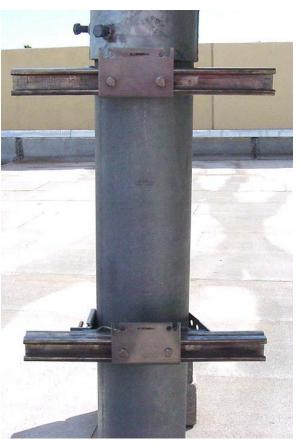
Figure B-6. Single-Thread with Hardware
