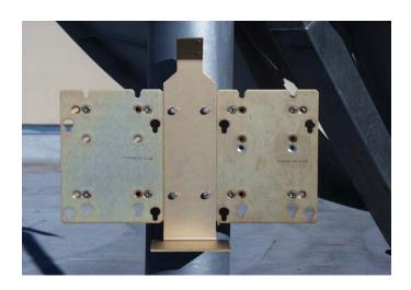
Figure A-18. Installation of Redundant Brackets
